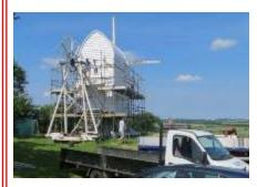
the tail assembly . The 1960's skeleton tail fan is unsafe and the the stairway need attention. Planning permission for both is imminent and our millwright, Bill Griffiths, aims to remove the tail carriage before the end of summer and rebuild it offsite.Bill also has to repair one of the sail frames currently in Chris Bates's barn and one of the main sail stocks still
