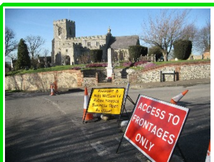
20 Feb -Nearly finished!
