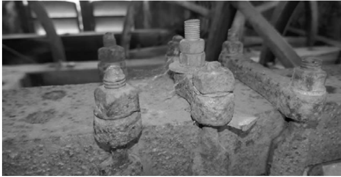
Bolts on top of No4 bell headstock – rusty and knurled with crude packing under one nut.
