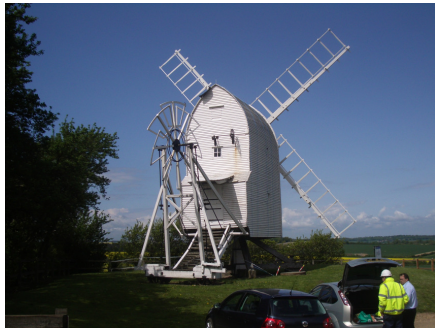
The Windmill being measured up for repair on 17 th May
