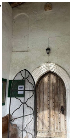
Filled porch doorway
