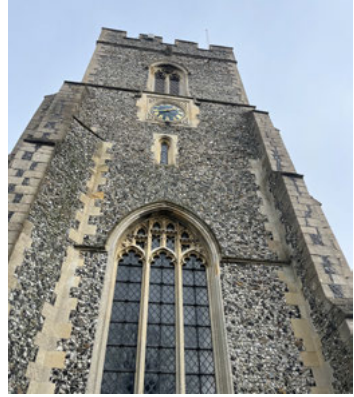
West Wall of Tower
